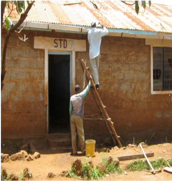
Erection of fisual board & gutters
