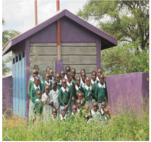
State of girl's latrine after renovation
