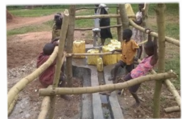
BOREHOLE WELL REPAIRS....
