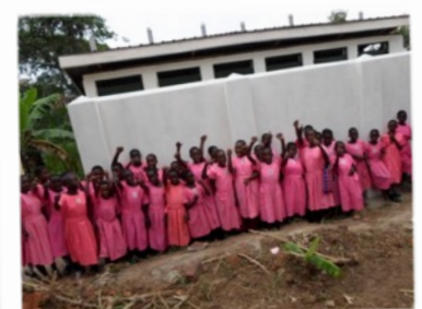
CANASSIST-FUNDED GIRLS LATRINE AT THE KAYENJE ELEMENTARY SCHOOL IN RURAL UGANDA.
